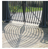
9 Gates & Fencing to Portishead Primary School Matthew Fedden
